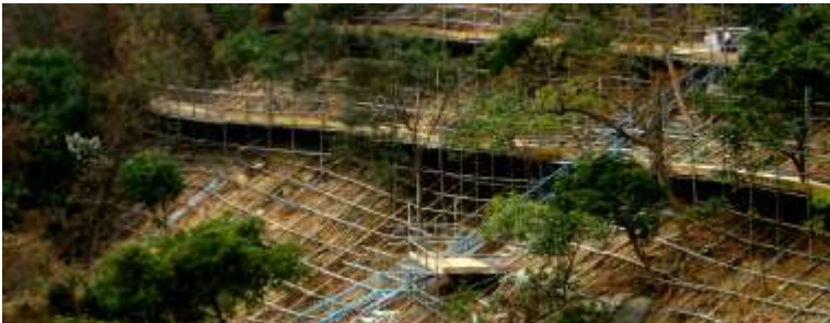
LPM works, CEDD Contract No. GE2003/26 slopes alongside Shing Mun Catchwater, Tsuen Wan - Government of HK SAR
