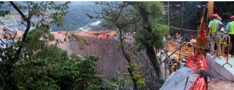
LPM works, temporary access road at Shatin Heights - China Railway
