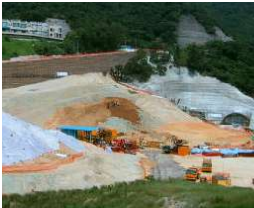
LPM works - Hong Kong
