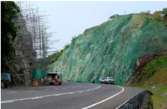
Slope stabilisation works for Bukit Kijal, Kemaman, Terengganu
