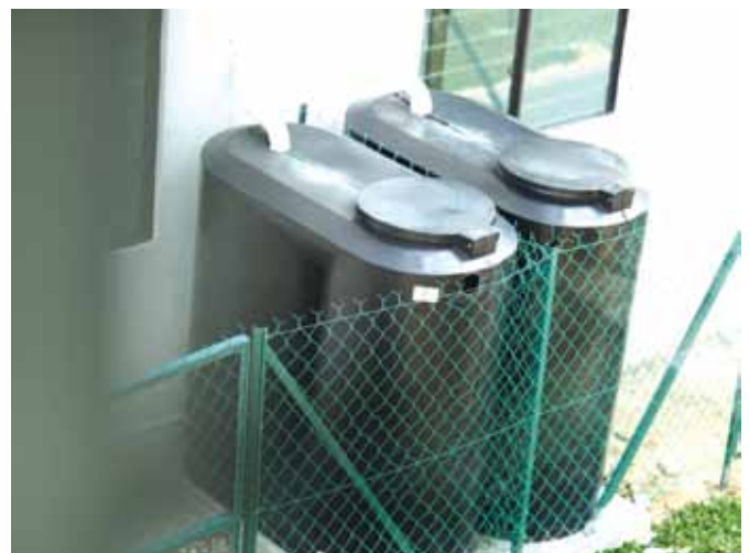
Rainwater harvesting tanks
