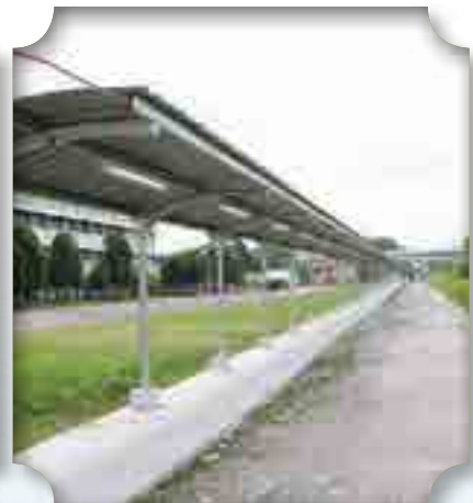
Provision of covered walkway to the commuter station
